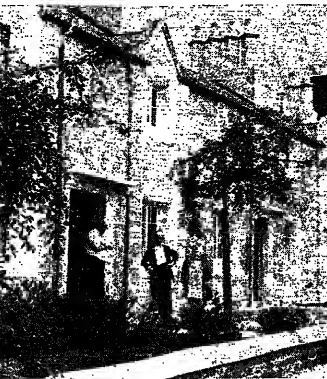
THE RESTORATION of a 19th-century railway workers' village in the centre of Swindon, Wiltshire, has received the accolade of the Royal Town Planning Institute, which this week presents its silver jubilee cup for environmental improvement to the local authority, Thamesdown.
